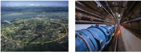
Figure 1 – CERN Large Hadron Collider ring and tunnel containing superconducting magnets for the guidance of the particle beams ( CERN Website, 2022 ).
